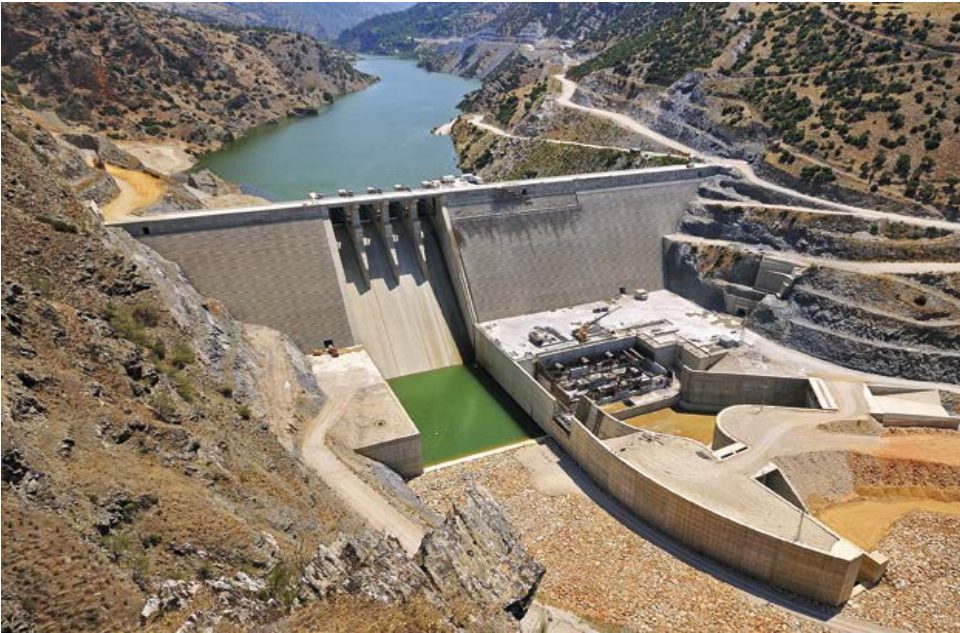
Cindere dam (H=107 m) in Turkey, the highest hardfill dam in the world
