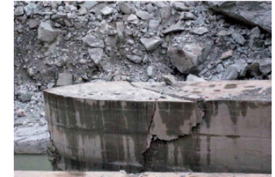
12, 2008 Wenchuan earthquake; Above right: Sheared off pier of Futan weir earthquake
