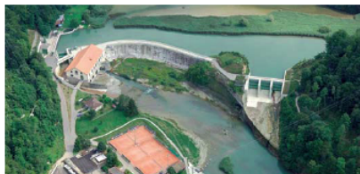
Left: Malgrange gravity dam built in 1872 in Switzerland. After a recent rehabilitation its service life has been extended by another 50 years. Photo shows the main elements of a storage dam for power production: spillway, reservoir, concrete dam body, power intake and powerhouse (left). Below from left to right: Downstream view of the 106 m high Sofid Rud buttress dam in Iran damaged by the magnitude 7.5 Marjil earthquake of June 21, 1990. Bottom: Intake outlets were opened after the earthquake to lower the reservoir (left). Rockfall damage near left abutment (middle) and right abutment (right).
