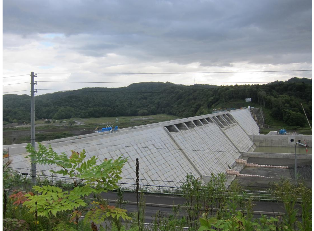
Tobetsu CSG dam (H=52 m) in Japan
