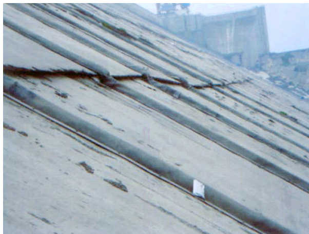
Figure 7 The overlapping of the second stage and third stage face slabs
