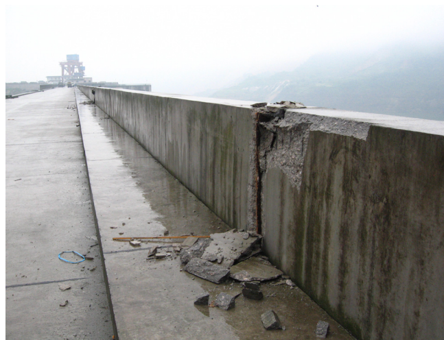
Figure 9 Rupture of parapet wall in riverbed section
