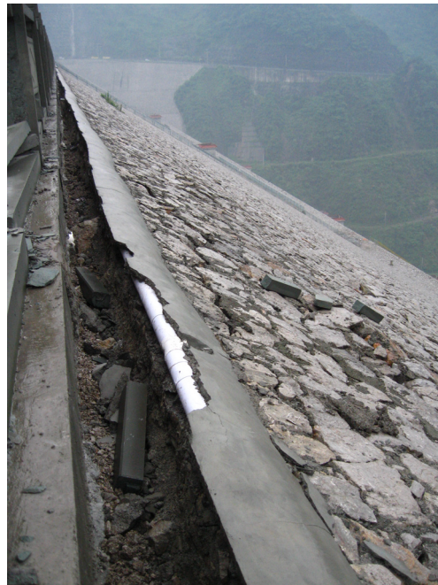
Figure 6 Crack at the downstream side of dam crest
