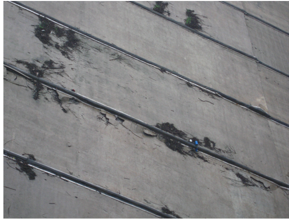
Figure 8 Rupture of concrete slabs along vertical joint
