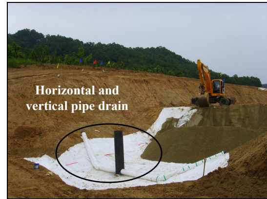
Fig. 5 Installation of the sand drain and filter mat at the toe of the embankment.
