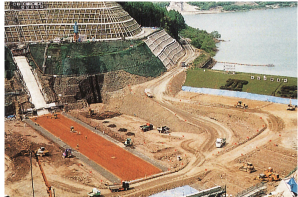
Photo 2 Raising Work of Embankment Dam (Sannokai Dam) 5)
