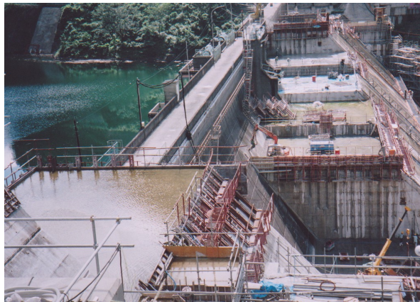
Photo 1 Raising Work of Existing Dam (Kayaze Dam) 3)
