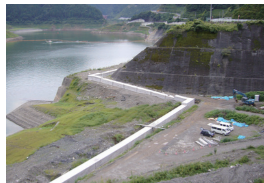
Fig.10 FRPM Pipe Section (2) (Completed with Concrete Cover)
