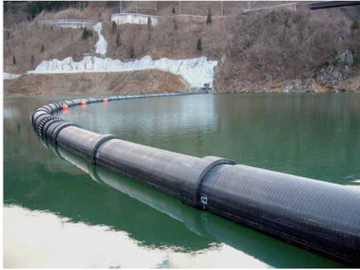
Fig.11 Suspended Pipe Section (1) (Before Submerging)
