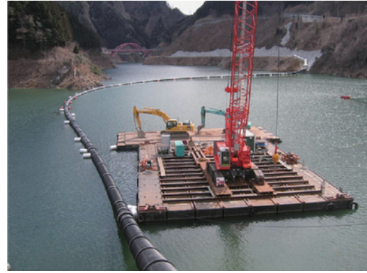
Fig.12 Suspended Pipe Section (2) (Construction Work)
