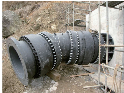
Fig.14 Suspended Pipe Section (4) (Rotation Joint)
