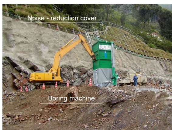
Photo 2. Installation of noise-reduction cover
