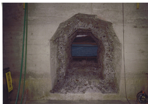
Figure-5 Dam body after drilling
