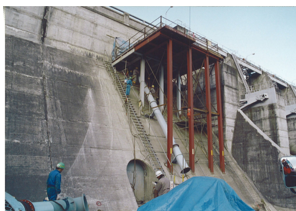
Figure-6 Installation works of outlet
